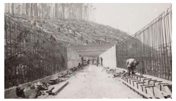
Figure 10: Construction of No. 1 Canal concrete flume section in the 1930s
