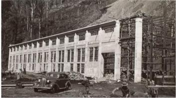
Figure 9: Construction of the powerhouse in the 1930s
