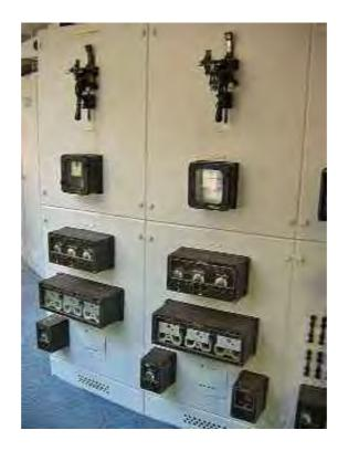
Figure 66: Relays and controls for the auxiliary generators. This is part of the only fully intact original generator system in the power station.
