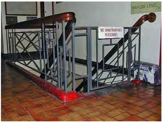
Figure 45: Central stairwell to first and ground floors showing late twentieth century tiled flooring and Art Deco painted welded steel balusters and gate, and varnished timber railing.
