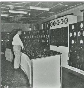
Figure 37: Control room in the 1960s. Note the additional dials and the change of lights from the original art deco style to fluorescent (HEC collection).
