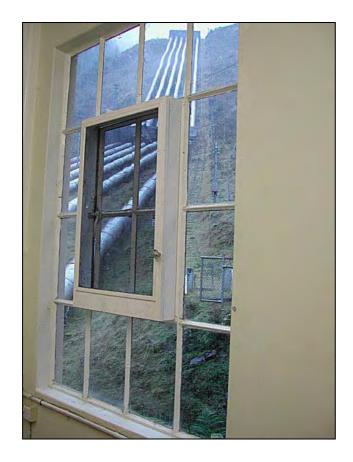
Figure 49: External window in team leader's office showing the centrally located opening casement and retro fitted timber framed insect screen. This window arrangement, with variation to the numbers of panes, is typical throughout the building.
