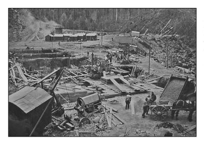
Figure 13: View of power station site in 1934/35 during earlier phase of construction showing the use of manual, horse driven and machine power (Cyril Young Collection, AOT -NS1938/138).
