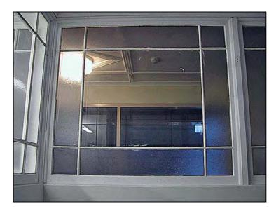
Figure 53: Internal window between S4 and passageway showing drawn glass central pane surrounded by *Belgian stippolite* perimeter panes. Note also the window to S3, the ceiling detail of the passageway and the smoke detector. The window arrangement is typical of the second floor internal windows throughout unless otherwise noted.
