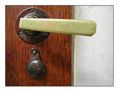
Figure 51: Detail of original door furniture in S4. This typical of many door handles found in the internal room doors on the second floor of the building.
