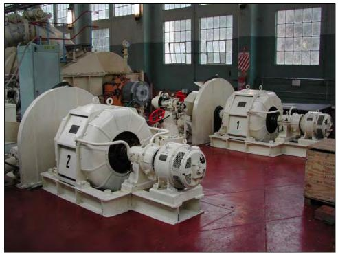
Figure 95: View of auxiliary (or 'house supply') generators 1 & 2. Exciters and turbines pictured.
