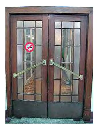
Figure 46: View of door between S1 and S2 showing timber and brass detailing, and both the plain and stippolite glass panels. Apart from the No Smoking sticker this door is identical to the door between S2 and S9.
