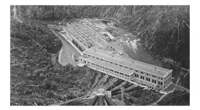
Figure 17: View of power station and switchyard soon after opening showing penstock, excavations for three more penstocks and the workshop/store adjacent to the switchyard (HEC collection).
