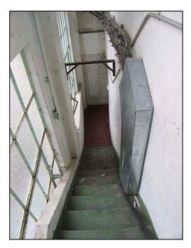
Figure 89: View of stairs, fuse box, cabling and windows with original window furniture including high window winding mechanisms.
