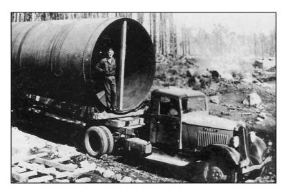
Figure 25: Section of 102 inch pipe being transported to hilltop penstock (HEC collection, reproduced in Marwood, p. 48).
