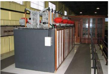
Figure 3.13 Circuit Breakers, Switch Gallery Waddamana A.
